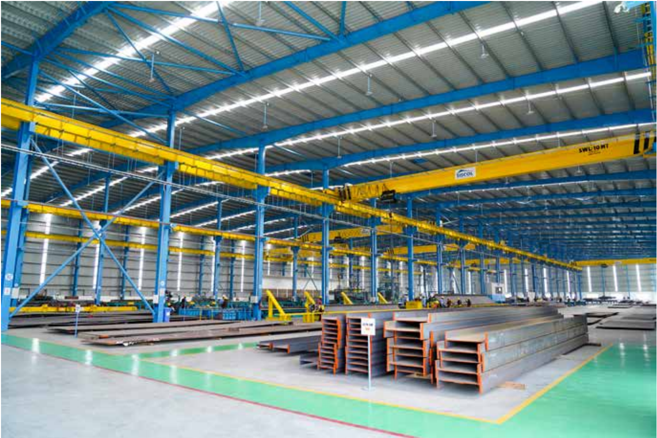
The inner view of the sparkling new Vadodara plant
