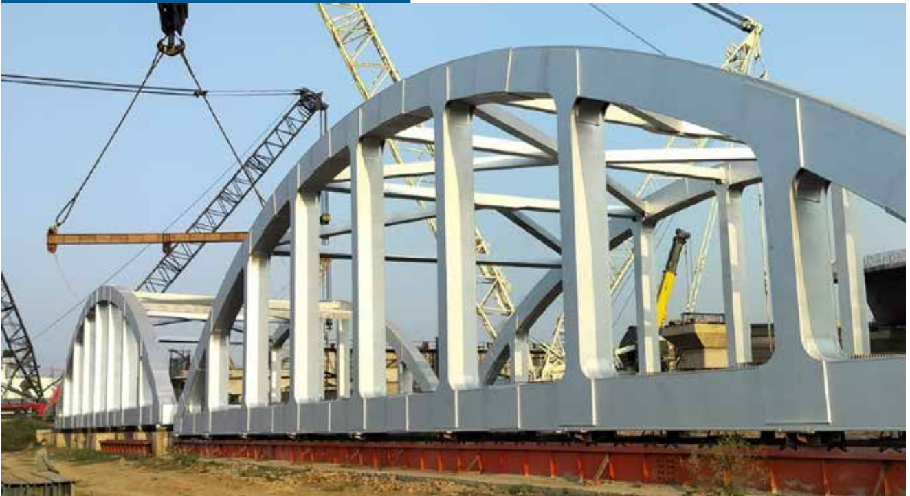
2x44m Bowstring bridge, final assembly stage
